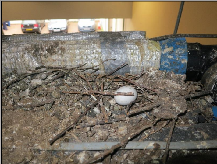
The cable trays above the car park of Dolphin Yard had become a nesting site for pigeons.
