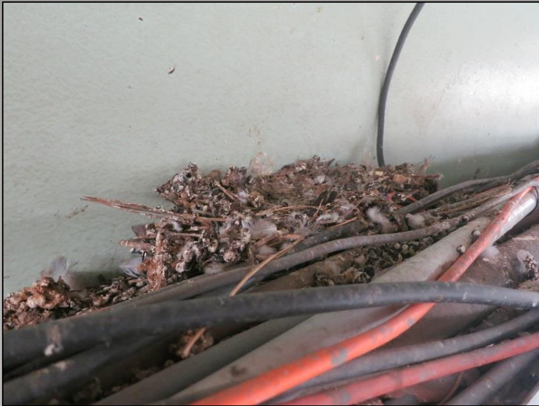
Pigeons were nesting and roosting in many of the high-level cable trays inside the factory.
