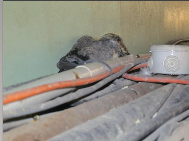
Pigeons were nesting and roosting in many of the high-level cable trays inside the factory.
